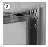
• Fix the frame to the wall through the holes in the canal.
